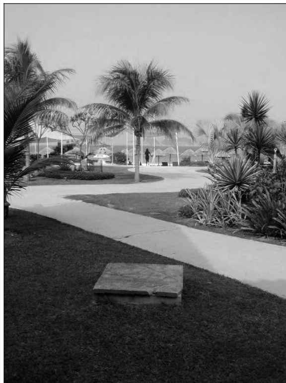
Figure 2. One of the groundwater wells contaminated by saltwater encroachment. The sea is located just beyond the end of the path.
